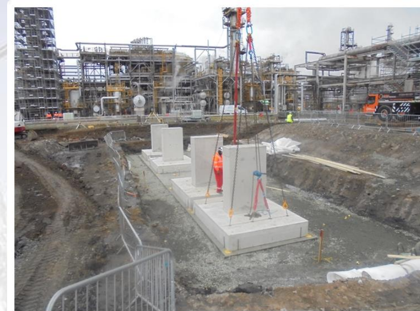
Staging manifold foundations being installed
