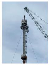
The new unit, which is proven in operation, uses Best Available Technology to ensure a clean flame but with the need for the addition of less steam – the main source of noise and vibration identified by our engineers.
