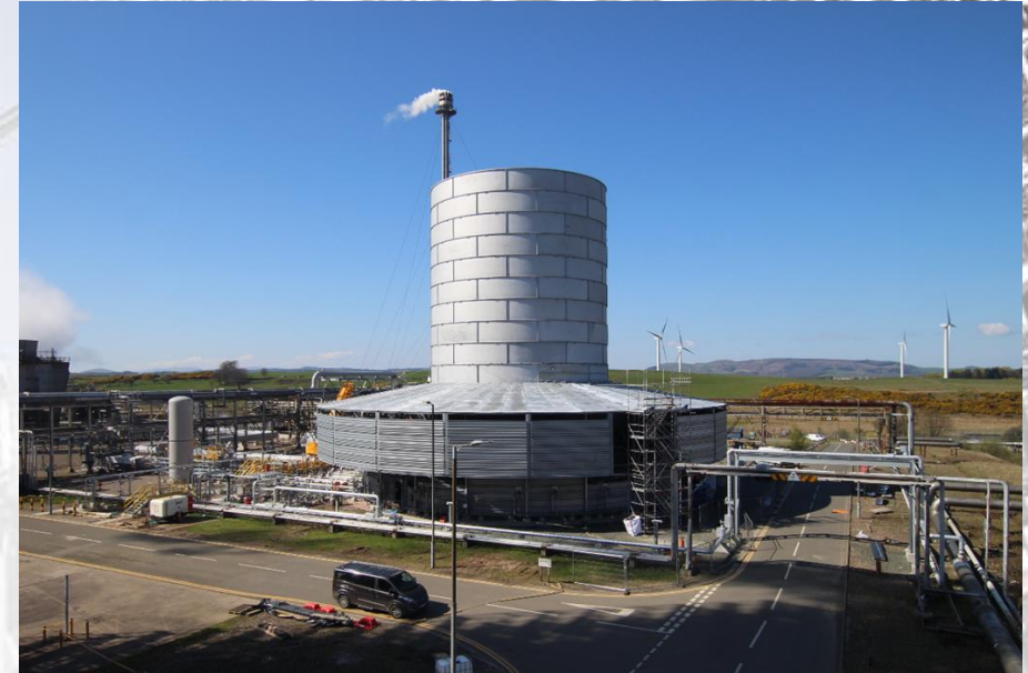
Panel installation nearing completion
