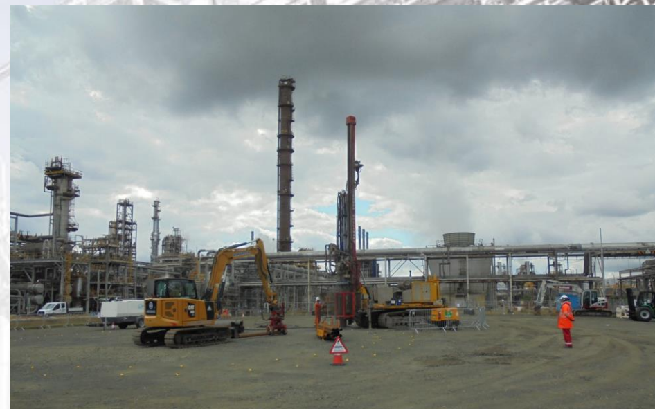
Phase 1 construction - ground piling continuing
