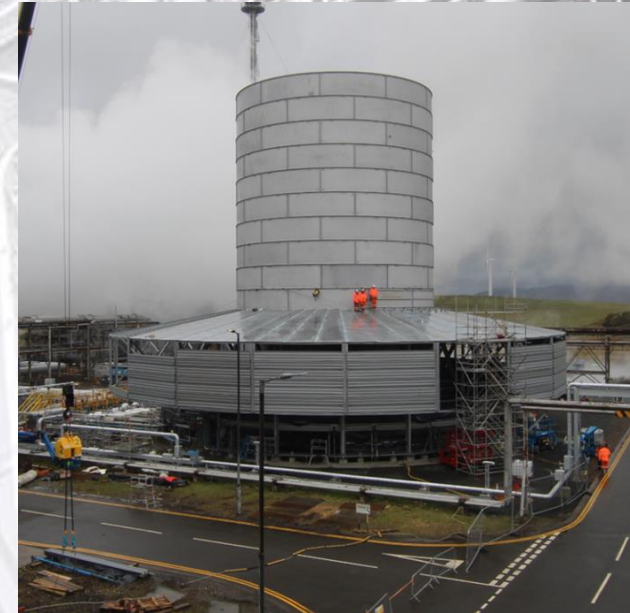
Upper and lower panel installation continues
