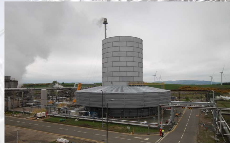
Shroud panel installation nearing completion
