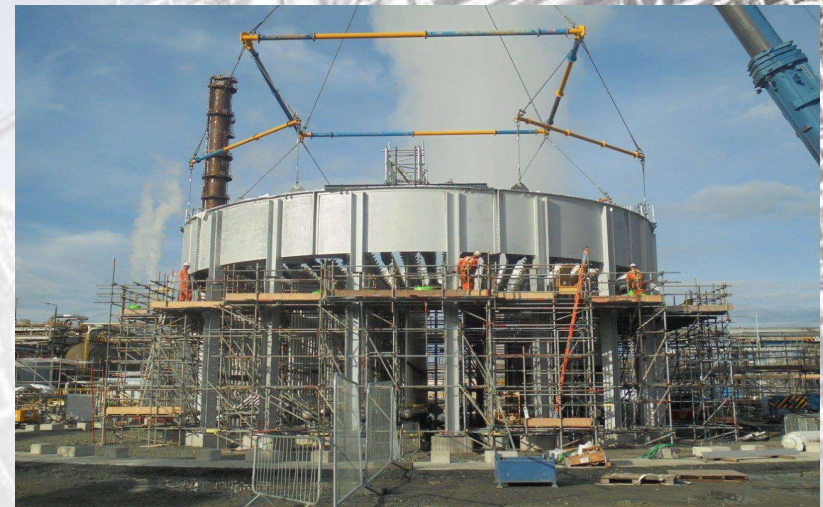
First EGF ring lift complete
