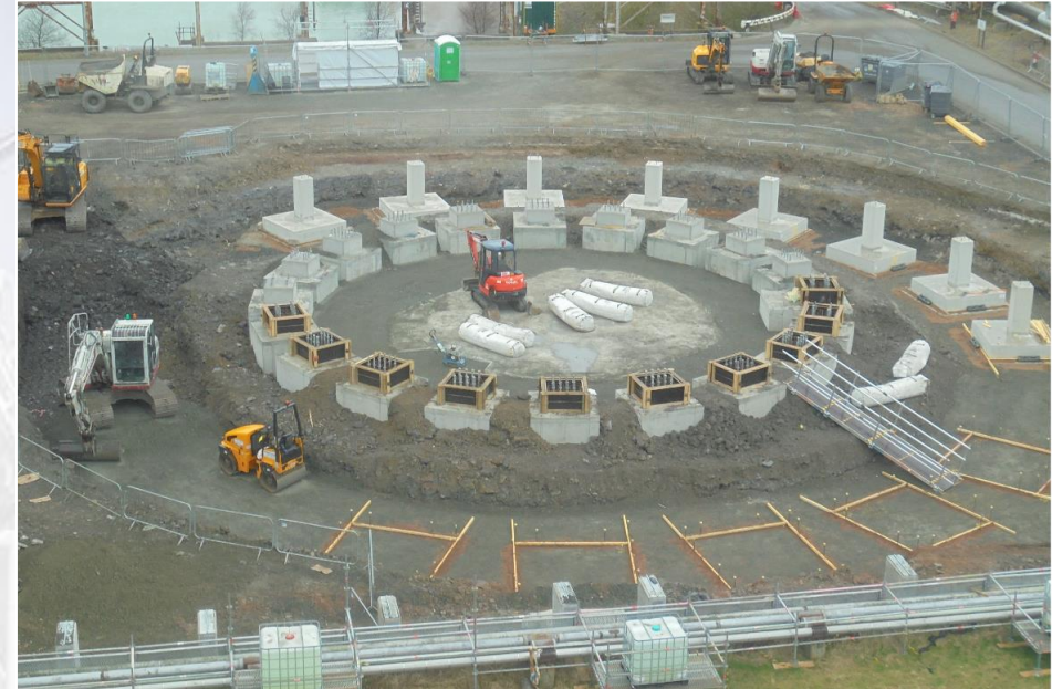
Pile Caps & Wind-fence foundation
