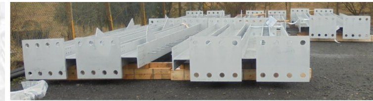
Structure beginning to arrive onsite at FEP
