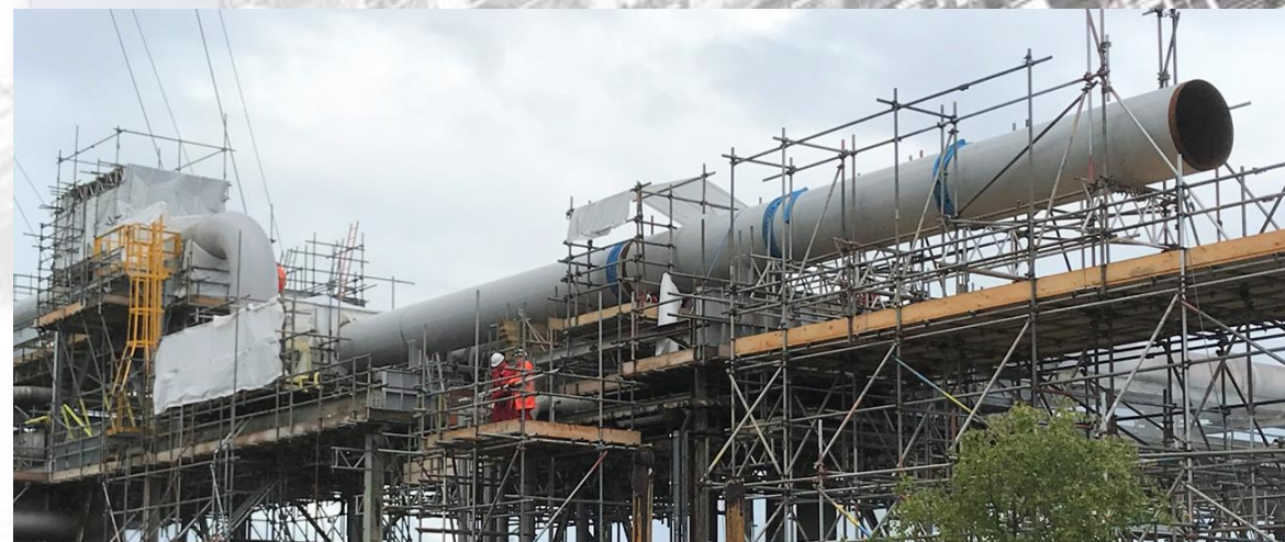
Flare header pipework installation progressing
